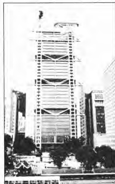
New HK & Shanghai Bank Headquarters — Argos' superior quality structural steel engineering work.
